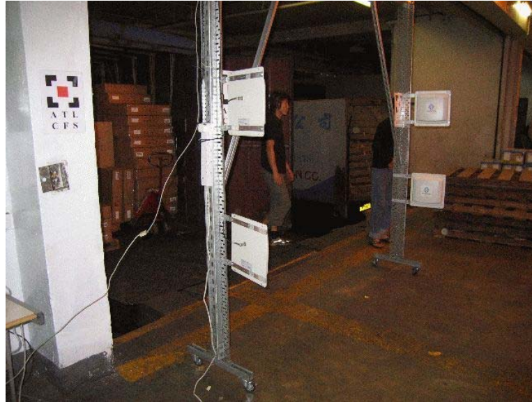
RFID Readers at Maersk Logistics Warehouse Gate In
