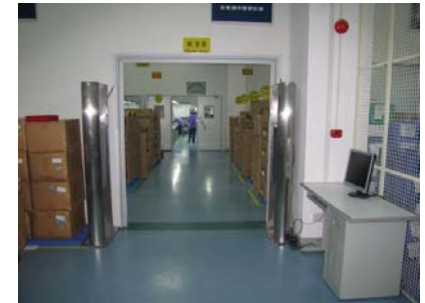
RFID equipment installed in the warehouse
